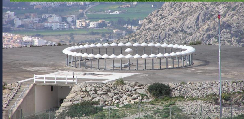
VOR/DME VHF omnidirectional range distance measuring equipment
