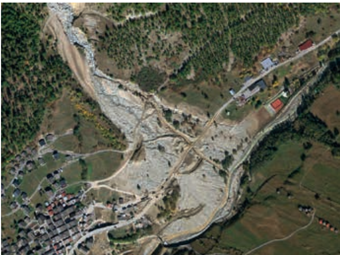
No damage assessment without reference data: aerial photograph of Wiler in the Lötschental (Canton Valais) before and after the storm in October 2011.
